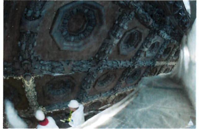
WORKERS PREPARE THE ROTUNDA'S COFFERED DOME FOR NEW PAINT.
