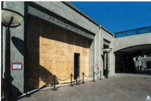
CAPITOL VISITOR CENTER EXTERIOR DOOR REPLACEMENT.
