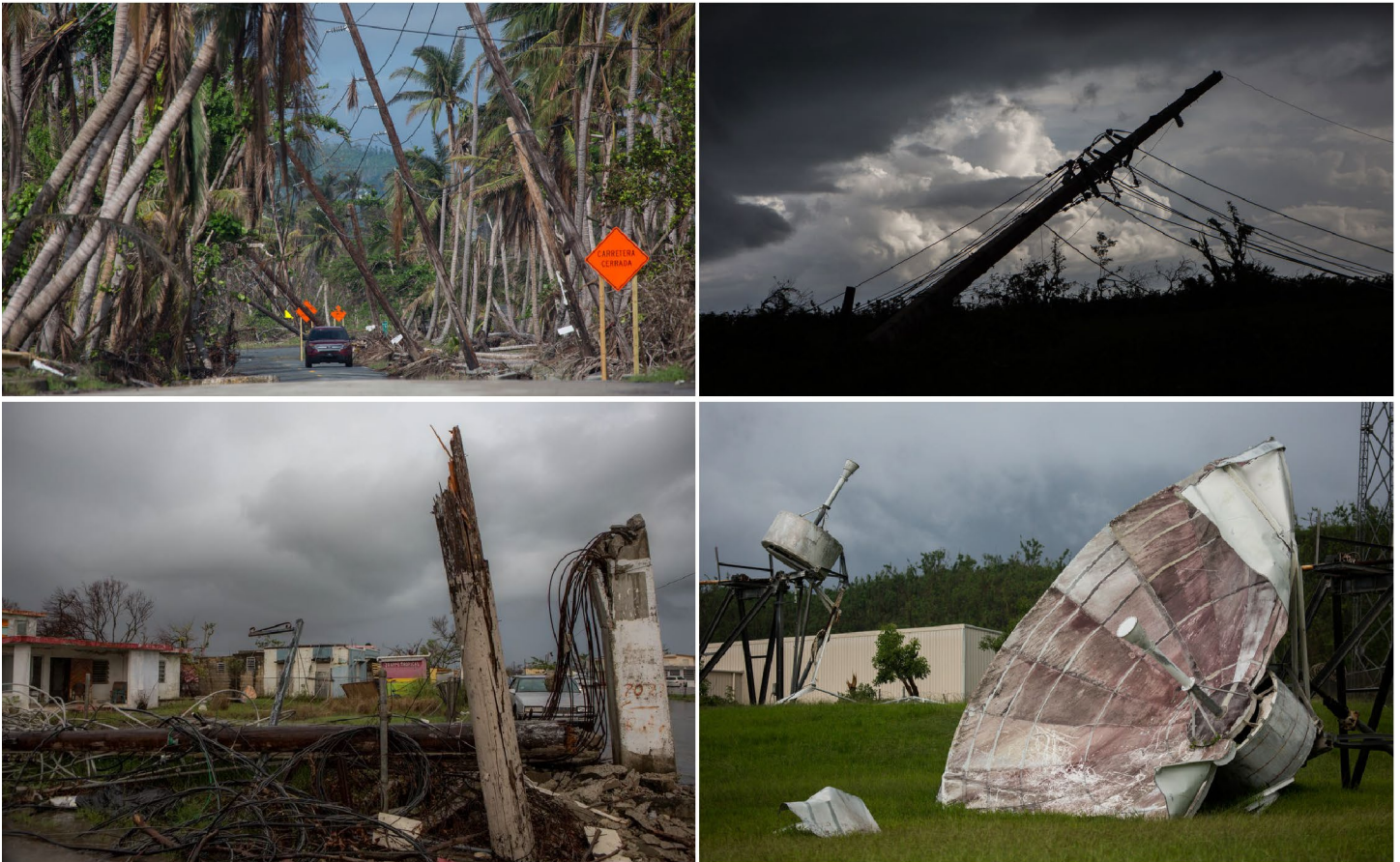
Figure 2: Damaged Power Lines and Satellite Dish in Puerto Rico after Hurricane Maria in November 2017
