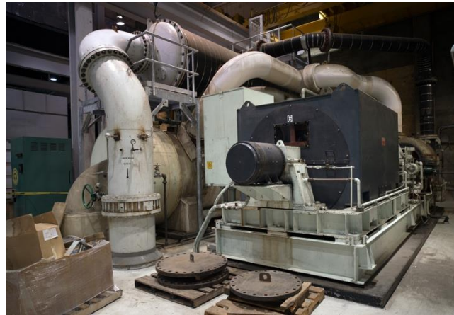
CAPITOL POWER PLANT REFRIGERATION PLANT REVITALIZATION PROJECT
