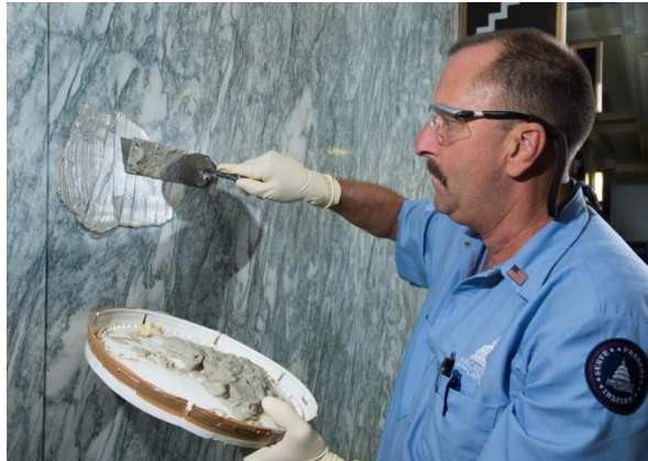
PERFORMING ROUTINE MAINTENANCE IMPROVES THE SAFETY AND SECURITY OF OUR INFRASTRUCTURE
