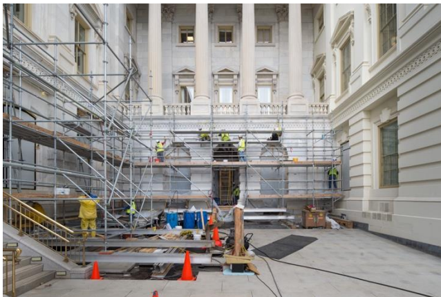
CAPITOL EXTERIOR STONE & METAL PRESERVATION PROJECT
