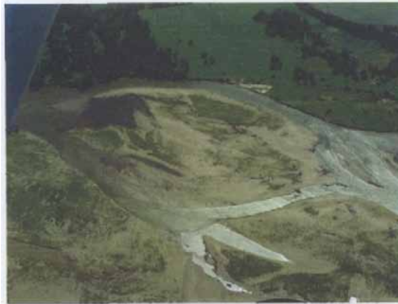
Existing sandbar and deadfall trees MR ~ 1308.5 Right Bank
