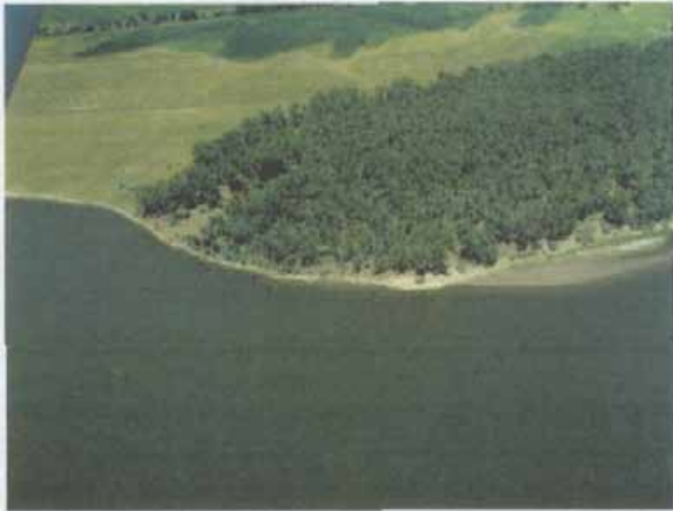
Southern End of Penitentiary Property Bank erosion and tree loss MR ~ 1308.5 Left Bank looking northeast
