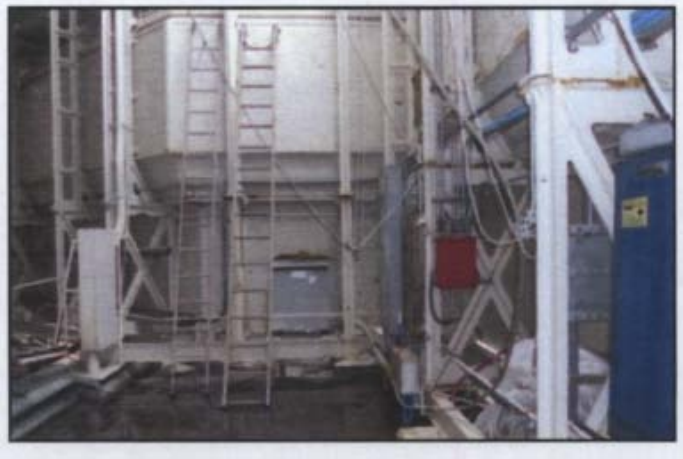
Interstitial space in the Capitol Dome.
