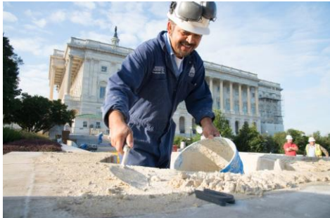
AOC stonemason makes repairs to the Olmsted Terrace Walls.
