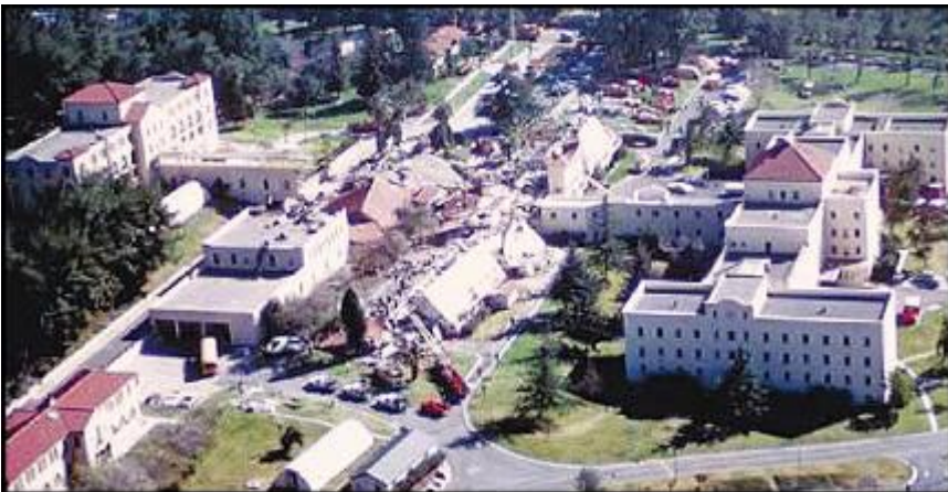
San Fernando Medical Center collapse, 1971
